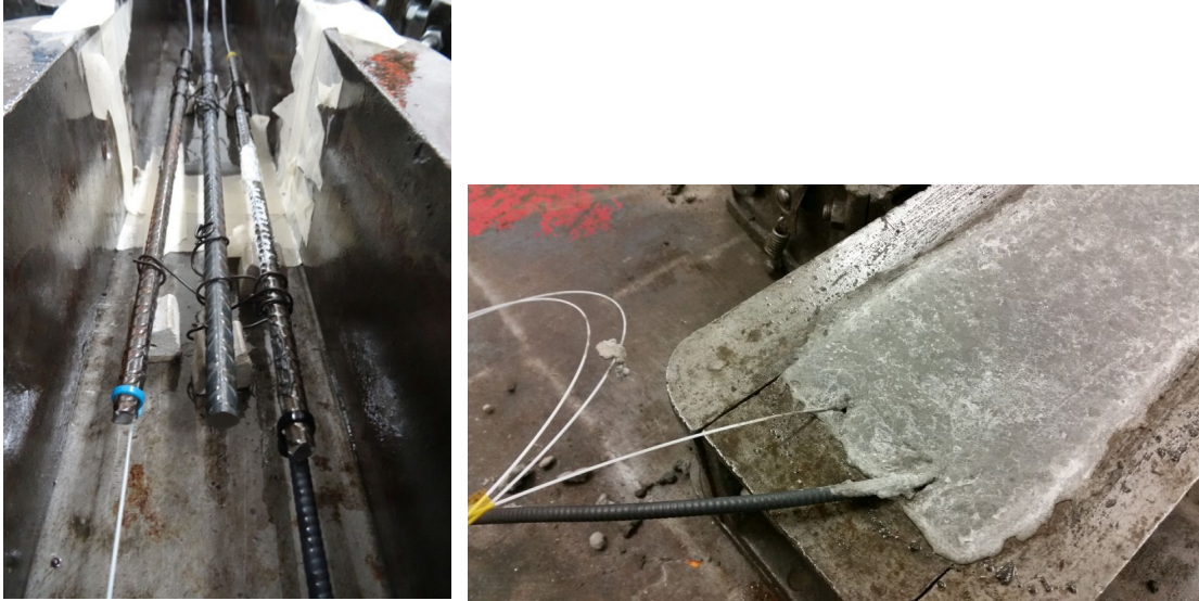
Fig.7. T130 GFRP-FBG cable sensor tied to reinforcement bar before pouring concrete.
